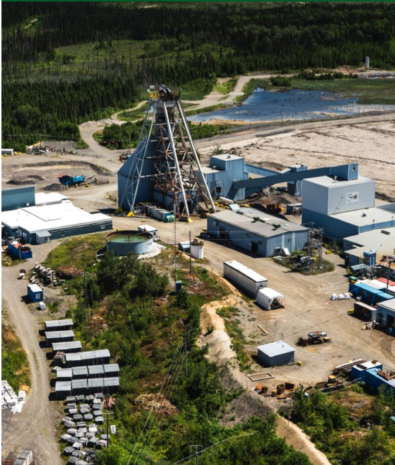
Bachelor Mill Complex (Mill, Tailings, Assay Lab & Camp)
